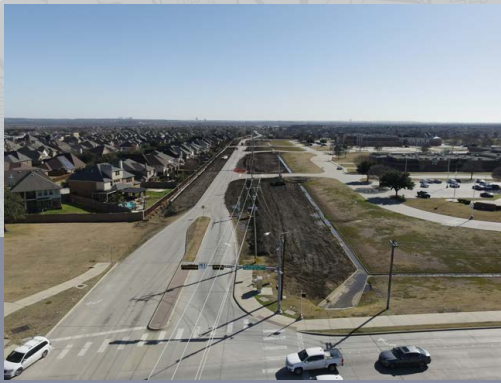
Day Miar Road clearing and grading looking south from Broad Street
