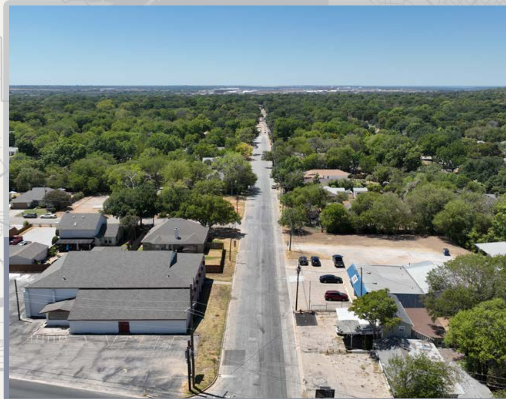
Barbara Road existing pavement looking west from Churchill Road
