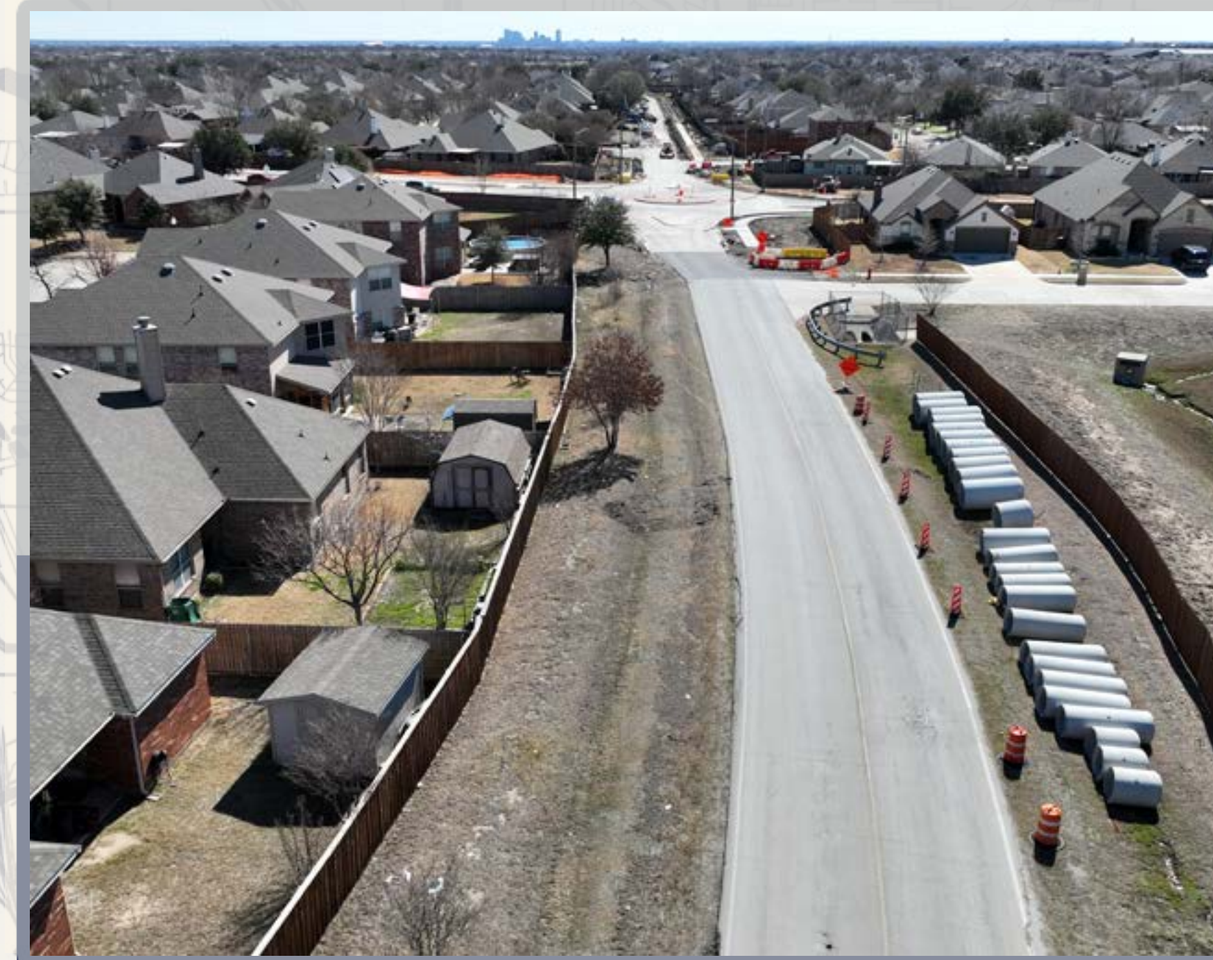
Knowles Drive during construction
