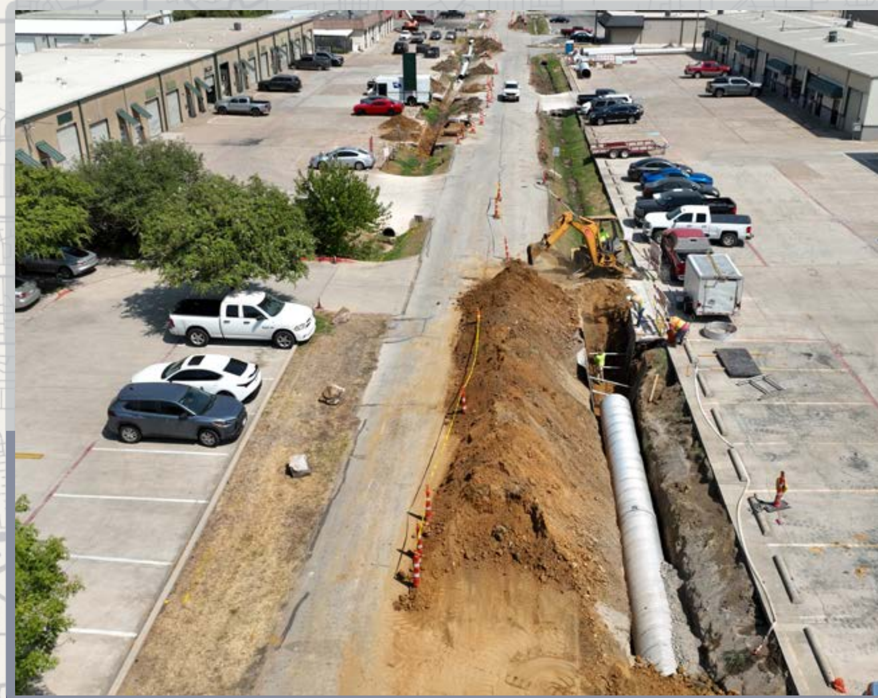
Construction of storm drainage system on Corzine Drive
