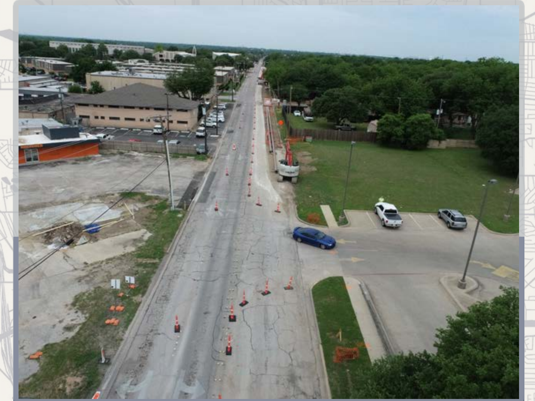
Construction of utilities along Glenview Drive
