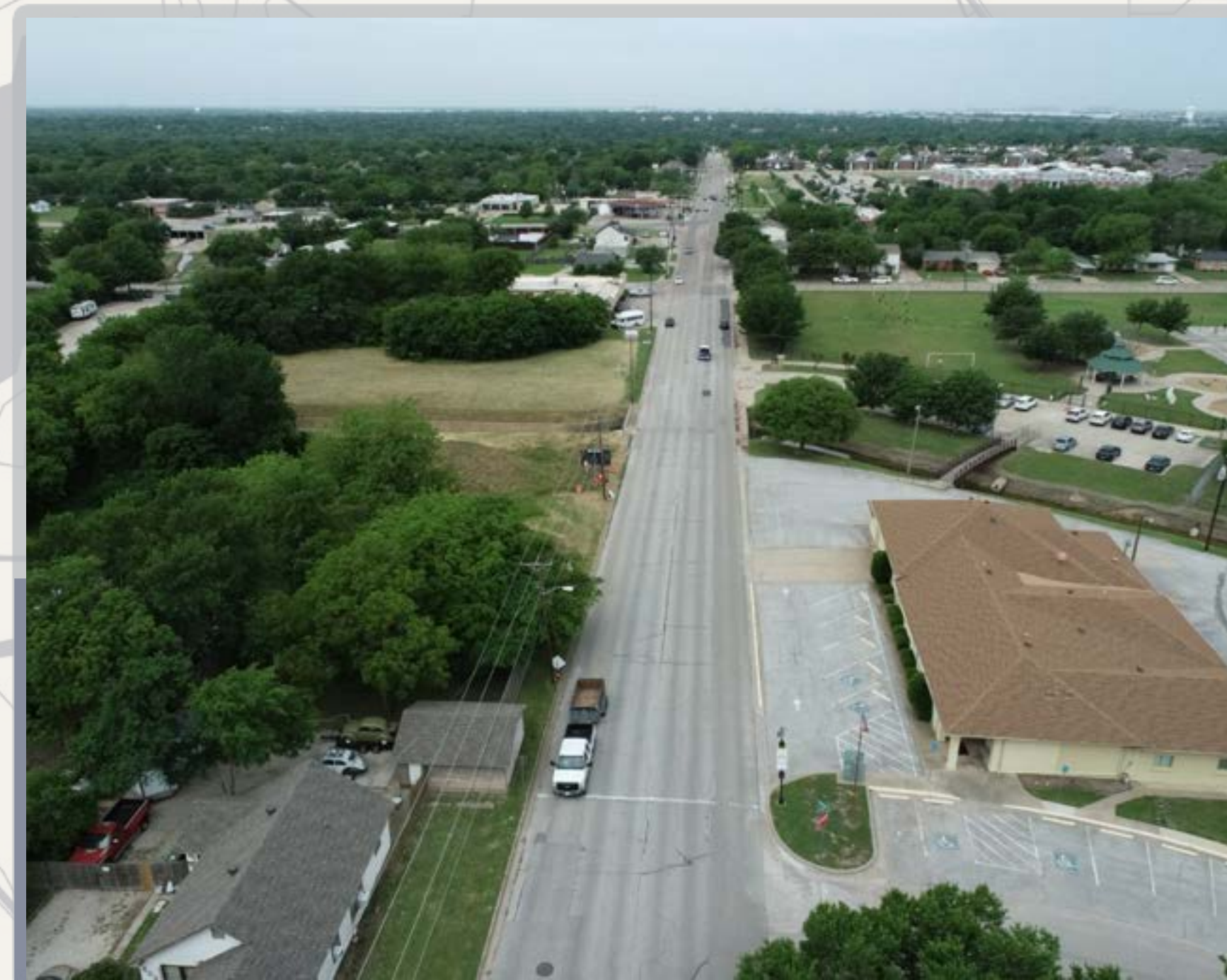
Glenview Drive prior to construction
