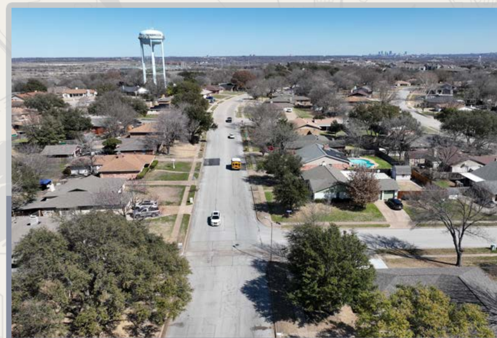
Reconstruction of Westpark Drive from RM 2871 to Lakeway Drive
