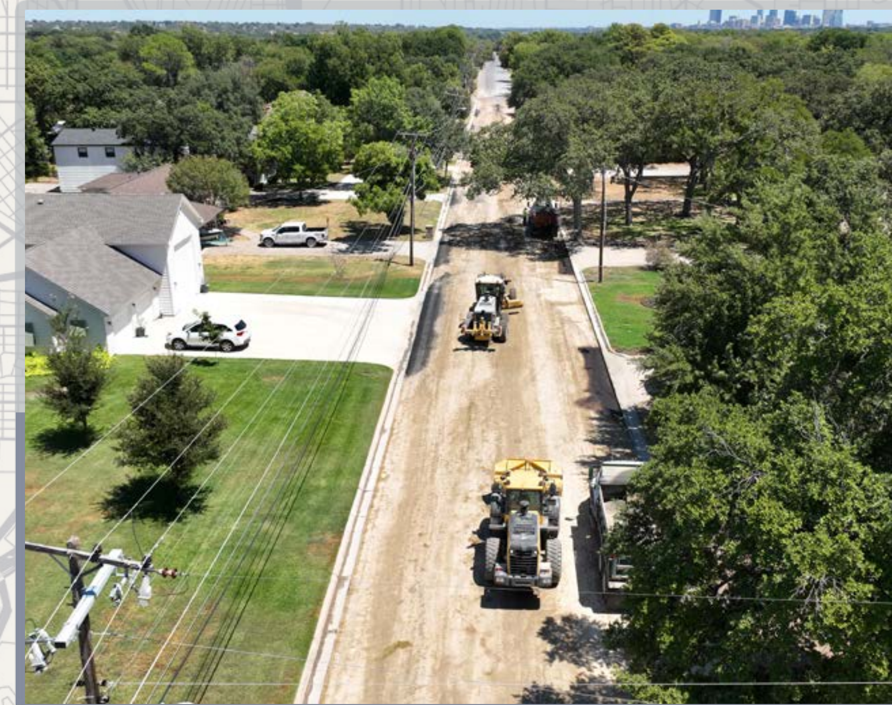
Current construction on Barbara Road
