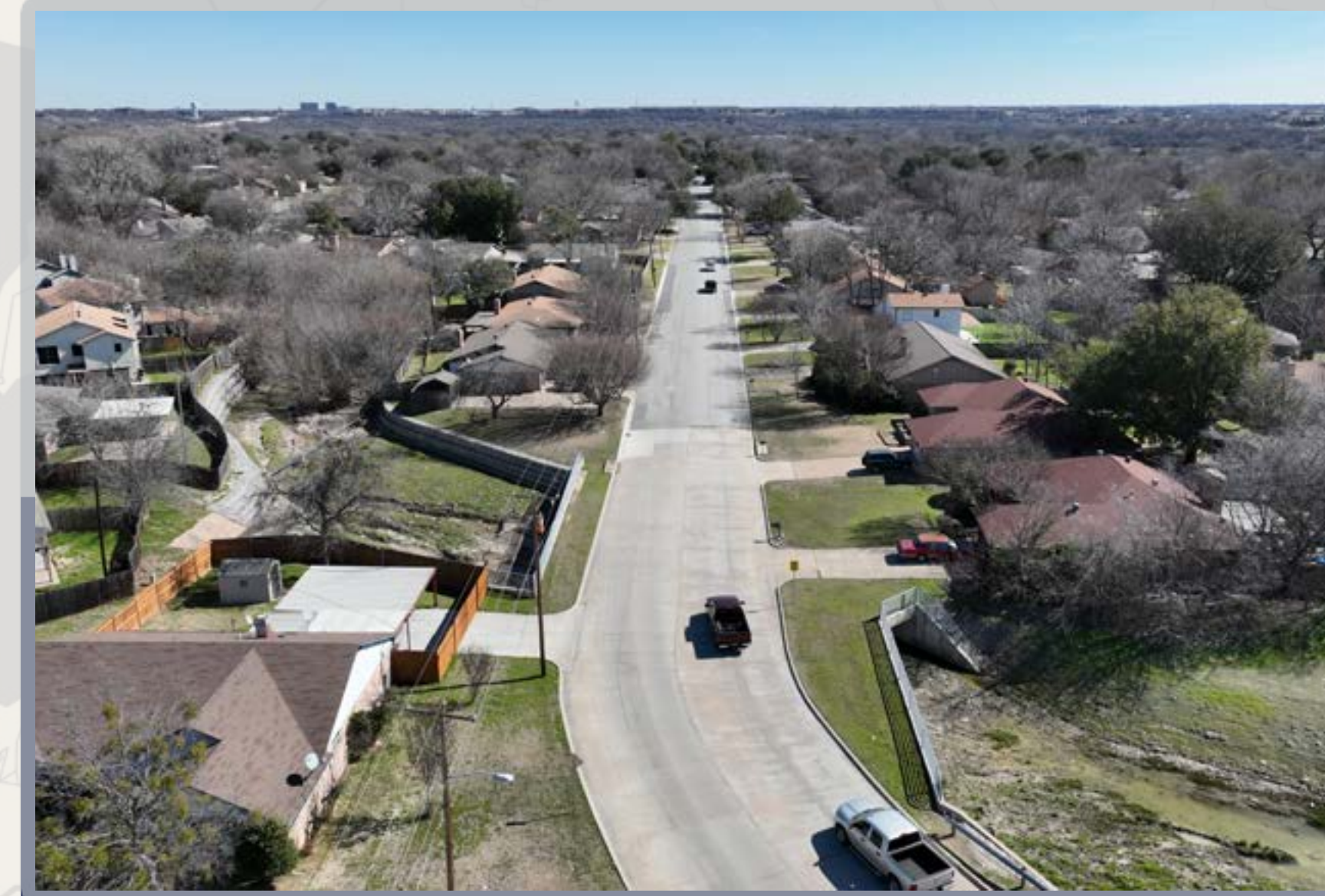
Reconstruction of Timbercreek Road from the bridge east of Winscott
