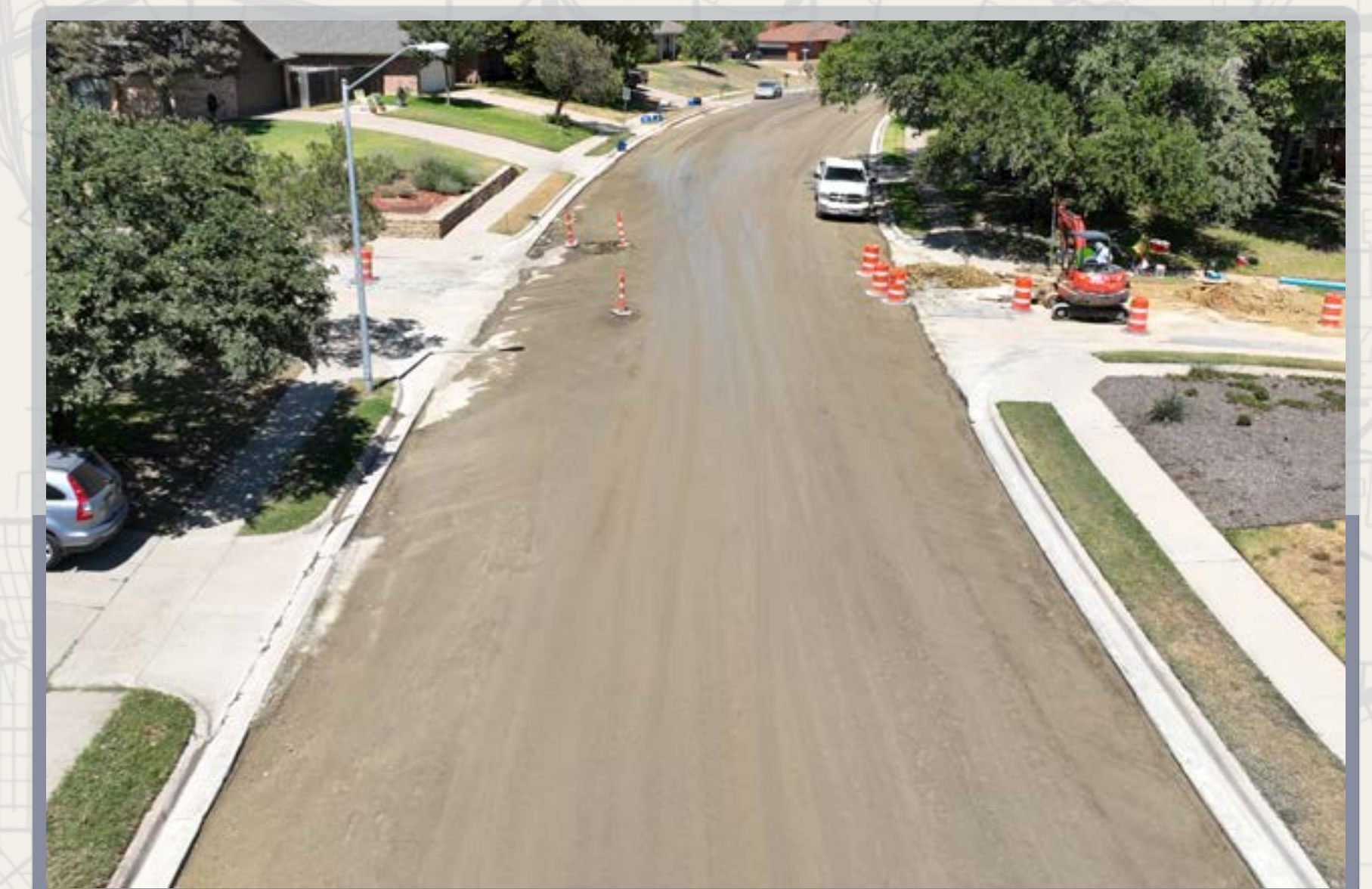
Westpark Drive under construction
